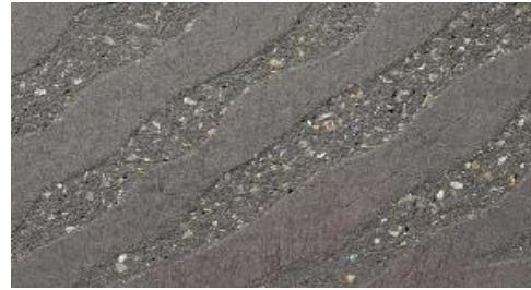
2 Concrete paving with sand blast finish.
